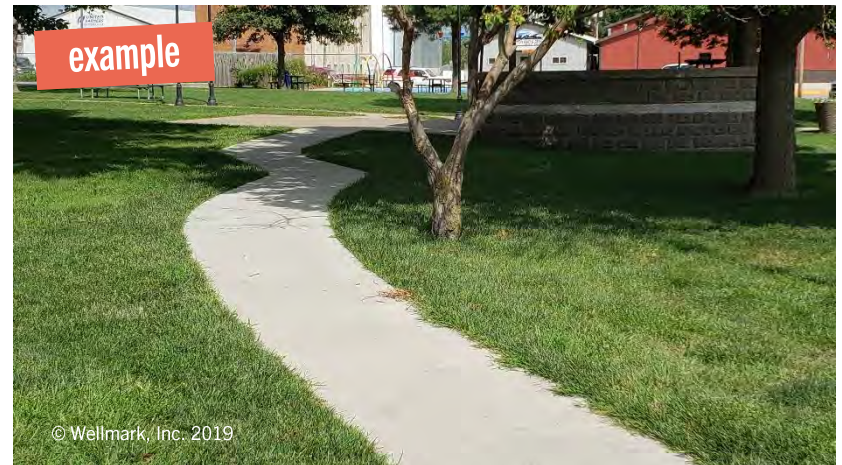
Example of a newly constructed sidewalk connection from Afton, Iowa.
