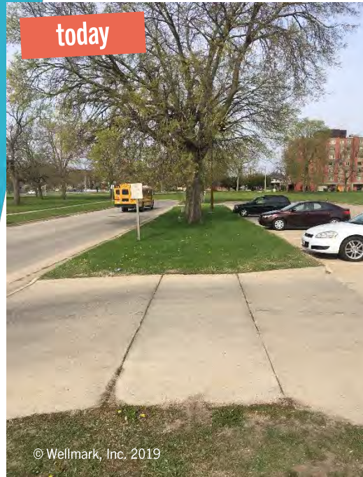
Areas of missing sidewalk like the one pictured above along Vine Street near East High School could be eliminated with the installation of infill sidewalk.
