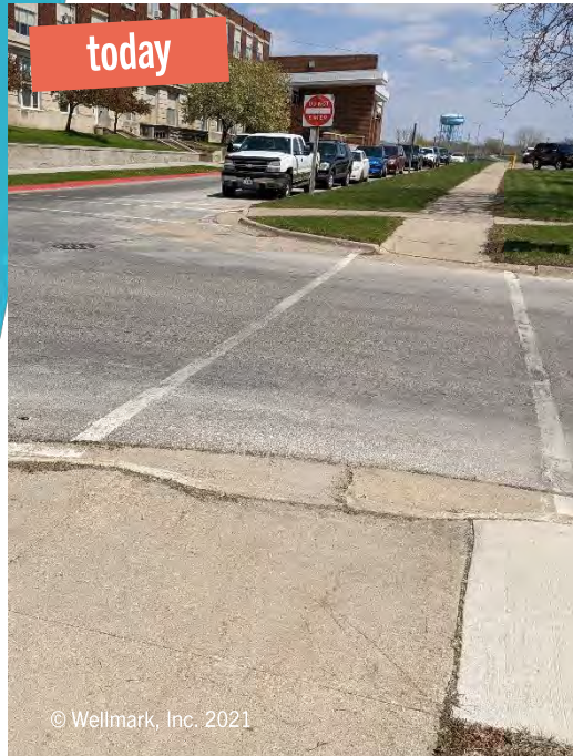
The curb ramps at this intersection need to be replaced to make them ADA-compliant.
