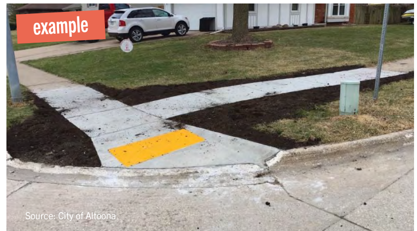
Example of a recently constructed ADA-compliant curb ramp from Altoona, Iowa.
