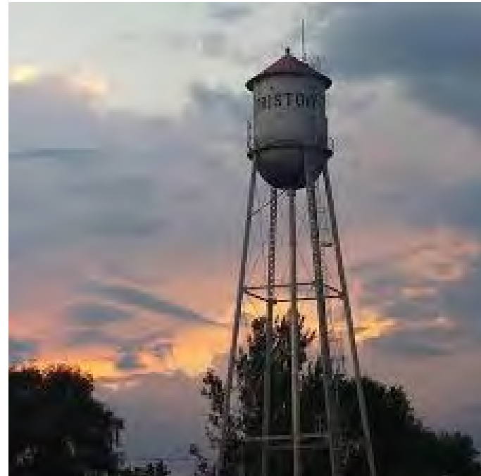
Bristow, Iowa Water Tower
